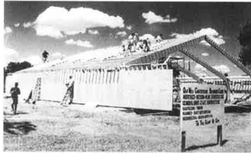
Farmington New Mexico church in progress
